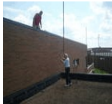
R-8 being mounted on the high school roof.
